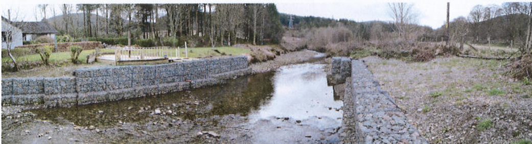
New weir/gauging station area
